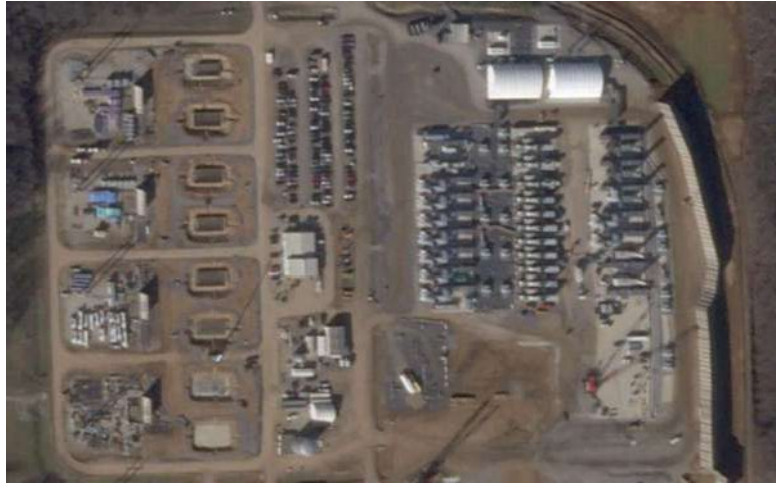
Figure 4. Close-up aerial image of xAI's Stanton Road S. facility showing 27 turbines (Feb. 9, 2026).
