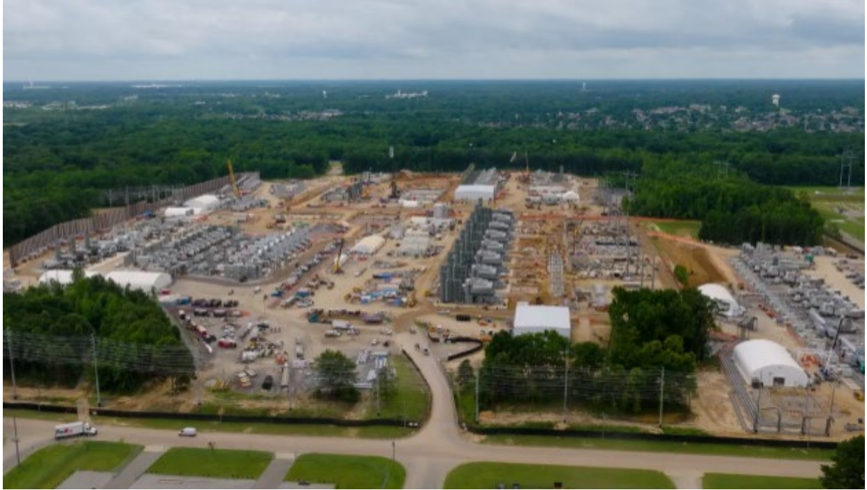
Figure 3: aerial image of xAI's Stanton Road S. facility (July 16, 2026)
